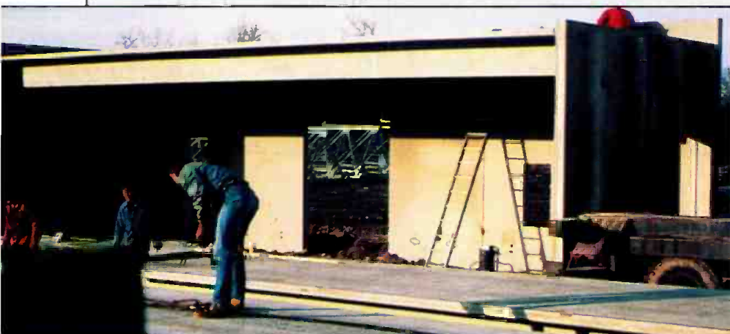
The transmitter building began to take shape during week 19 of the project. Precast wall panels were trucked to the site and lifted into place by a crane. At this point in the project, the local utility company had placed the necessary power poles and lines for ac service.
