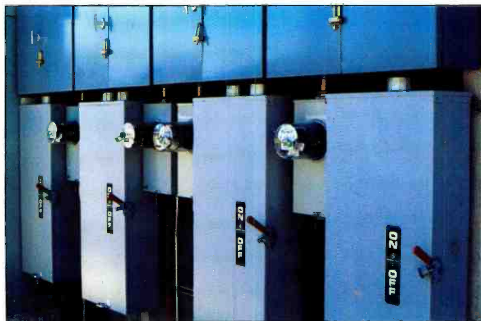
Each station in the complex has its own ac power watt-hour meter and service disconnect switch located outside the building. This switchgear and a nearby surface-mounted utility company transformer are protected from falling ice by heavy metal grating.
