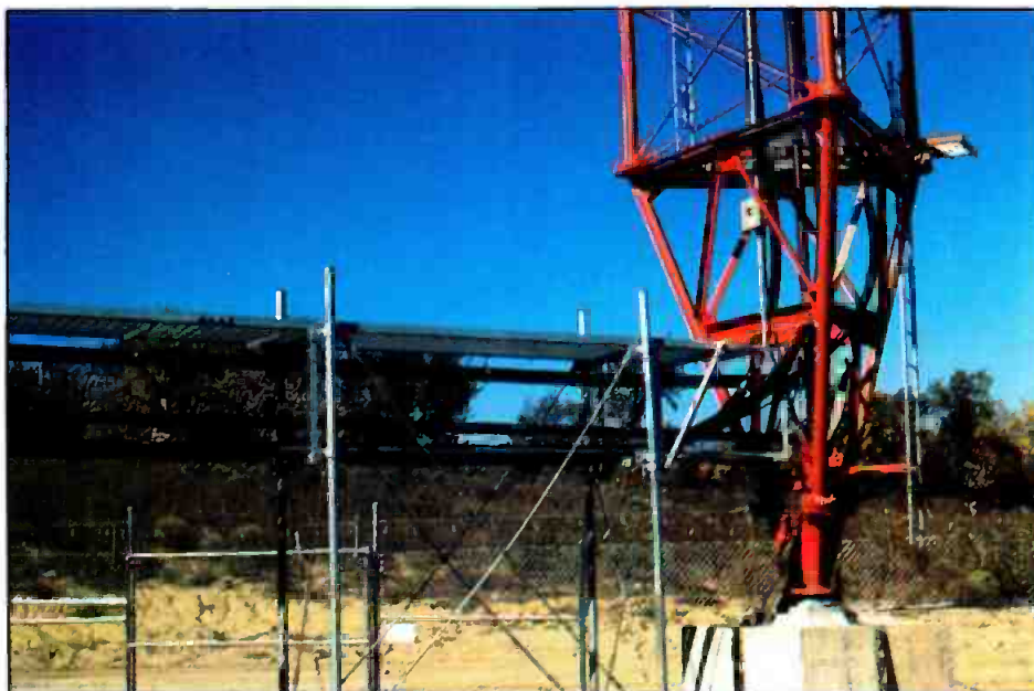
Grounding is a major concern for the transmitting tower because of the frequency and severity of lightning storms in the Kansas City area. The ground system consists of radials spread out from the base of the tower in a manner similar to an AM antenna ground. The transmission line bridge from the building to the tower can be seen below the ice shield.
