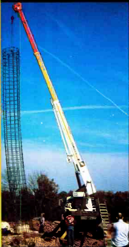
By week 10 of the project, the tower pier had been drilled and the rebar set in place. A 5-foot-diameter hole was drilled 56 feet down for the foundation of the structure.
