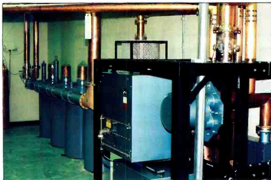
Cavity filters (shown in the background) are used on the output of each transmitter at the facility to prevent intermod problems. The combiner for the twin 25kW FM transmitters is shown in the foreground.
