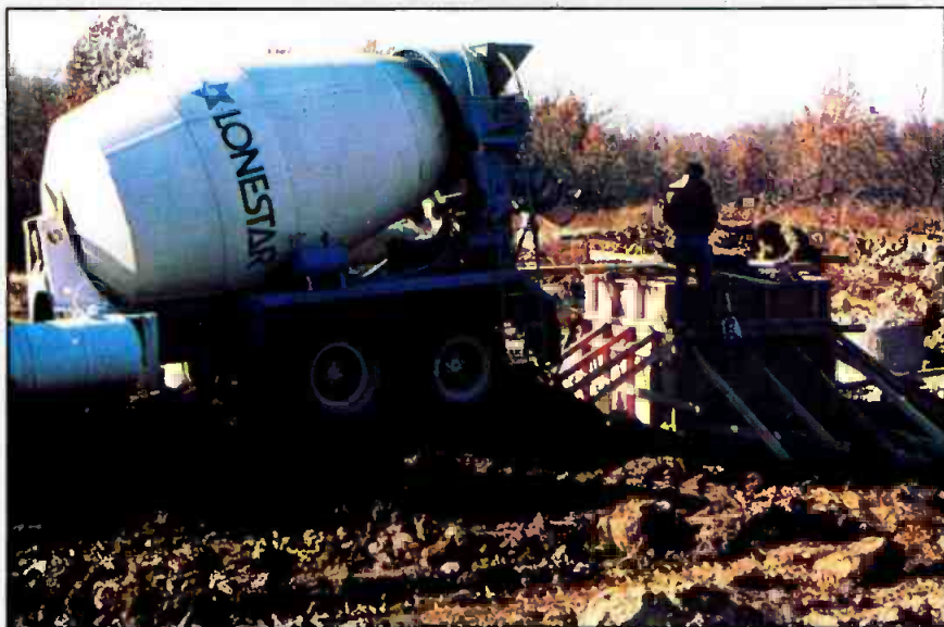
Concrete was poured at the tower base during week 12. At the same time, drilling was under way for the guy anchor posts. Some of the posts were drilled to a depth of 80 feet to ensure a sound footing and to avoid problems with the underground limestone mine.
