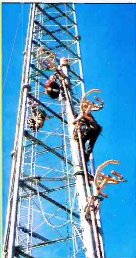
The top-mounted KLSI-FM antenna was hoisted up the tower on Feb. 7, 1987, week 24 of the project. At this point in the effort, electrical service for the transmitter building was well on the way to completion.
