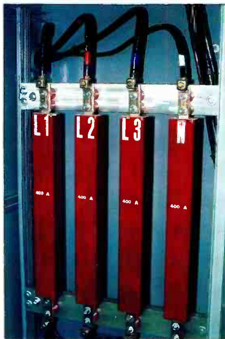
Transient protection is a major concern because of the high level of lightning activity. This transient suppressor protects the KLSI section of the facility.
