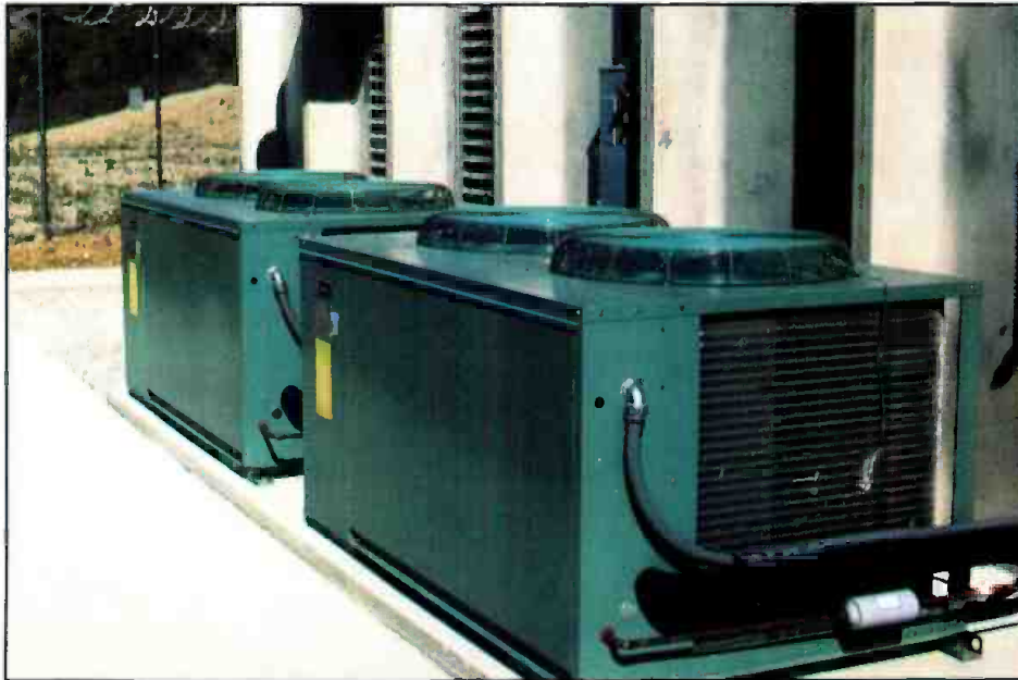
Two of the four stations have closed-loop cooling systems in which no outside air is used to cool the transmitters. Exhaust air from each transmitter is dumped into the room and large air-conditioning units are used to keep the rooms cool. The heat exchangers for one of the transmitter rooms are shown.
